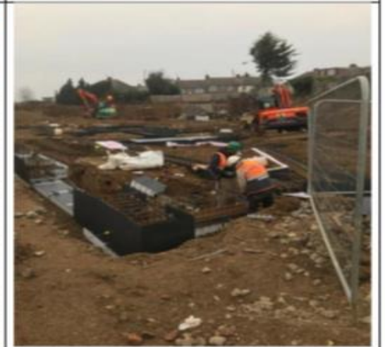
Description: Plot 53 – Ground beams
