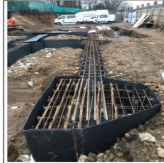
Description: Plot 53 – Block B Ground Beams
