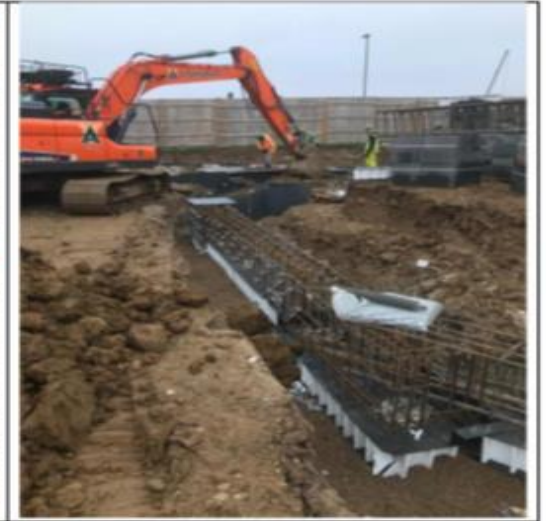
Description: Plot 53 – Block A Ground Beams
