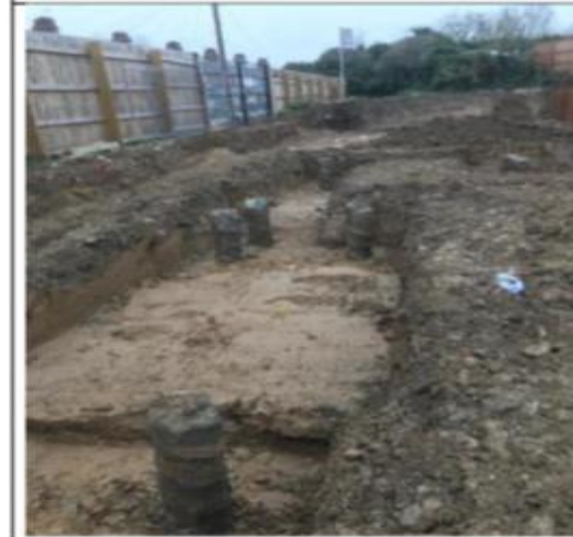
Description: Plot 54 – Block C Ground Beams
